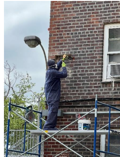
Masonry probe at Building 5
