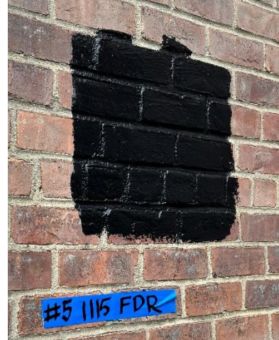
Waterproofing membrane installation for Adhesion Testing
