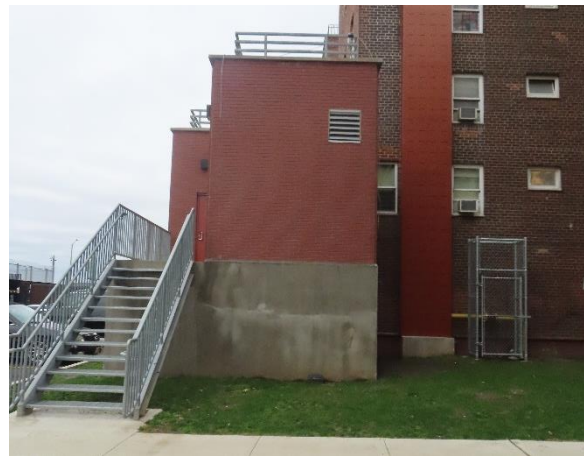
ATS at Building 4
