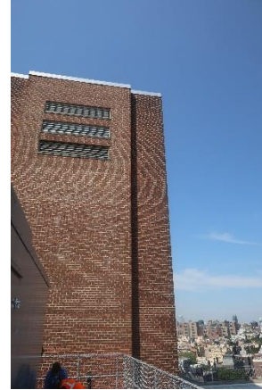
Water Tower at Building 11
