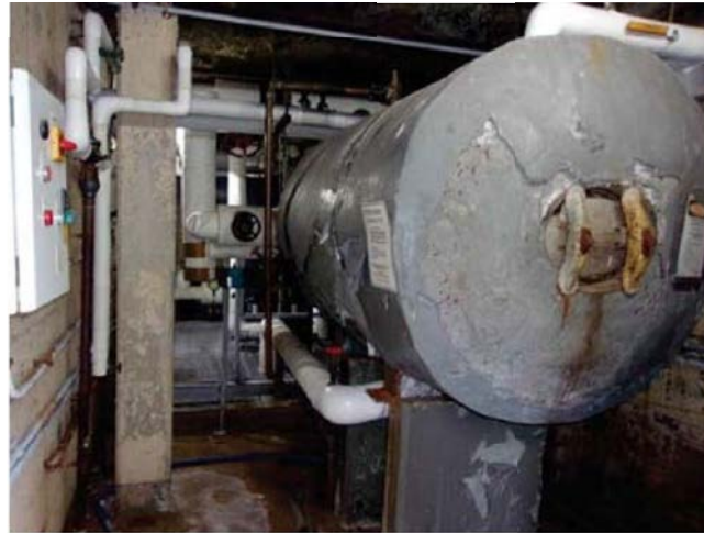
Steam to water generator and hot water storage tank system in Building 9
