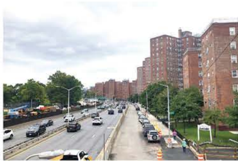
FDR Drive (Looking South)
