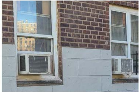
Flood Protection at Riis Houses
