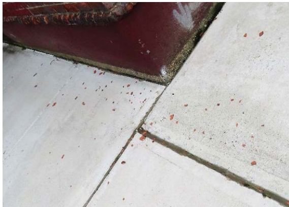
Pieces of brick spalls on the sidewalk
