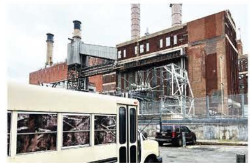
Con Edison East River Generating Station
