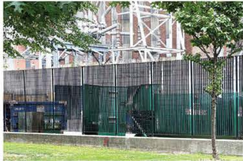
North Trash Compactor
