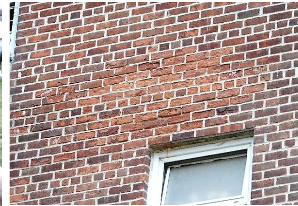
Building 2: Spalled brick at bathtub area
