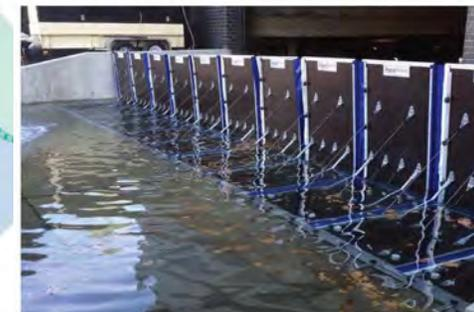
Example of Flood Planks Installed to Control Flooding
