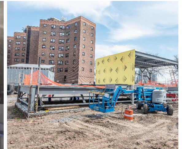
Mechanical Electrical Addition building under Construction
