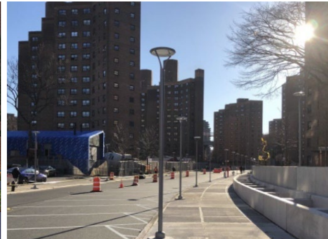
Baruch Drive – under construction
